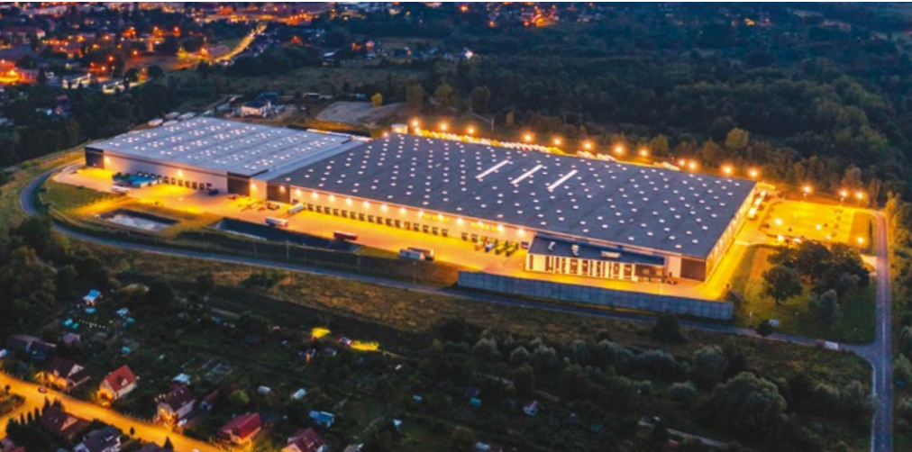
Lubuskie 2 Building, located in Krosno (Poland), had a building extension constructed in June 2023.
